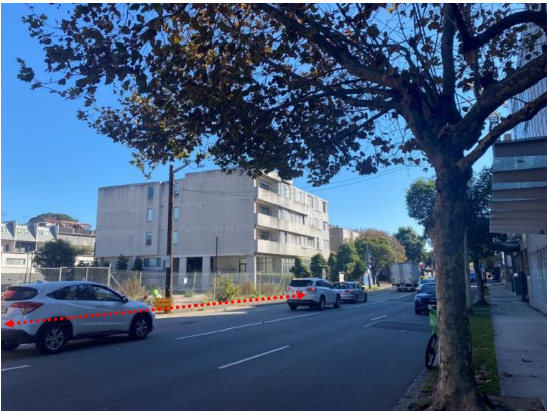
Figure 4: Looking north along Botany Road
