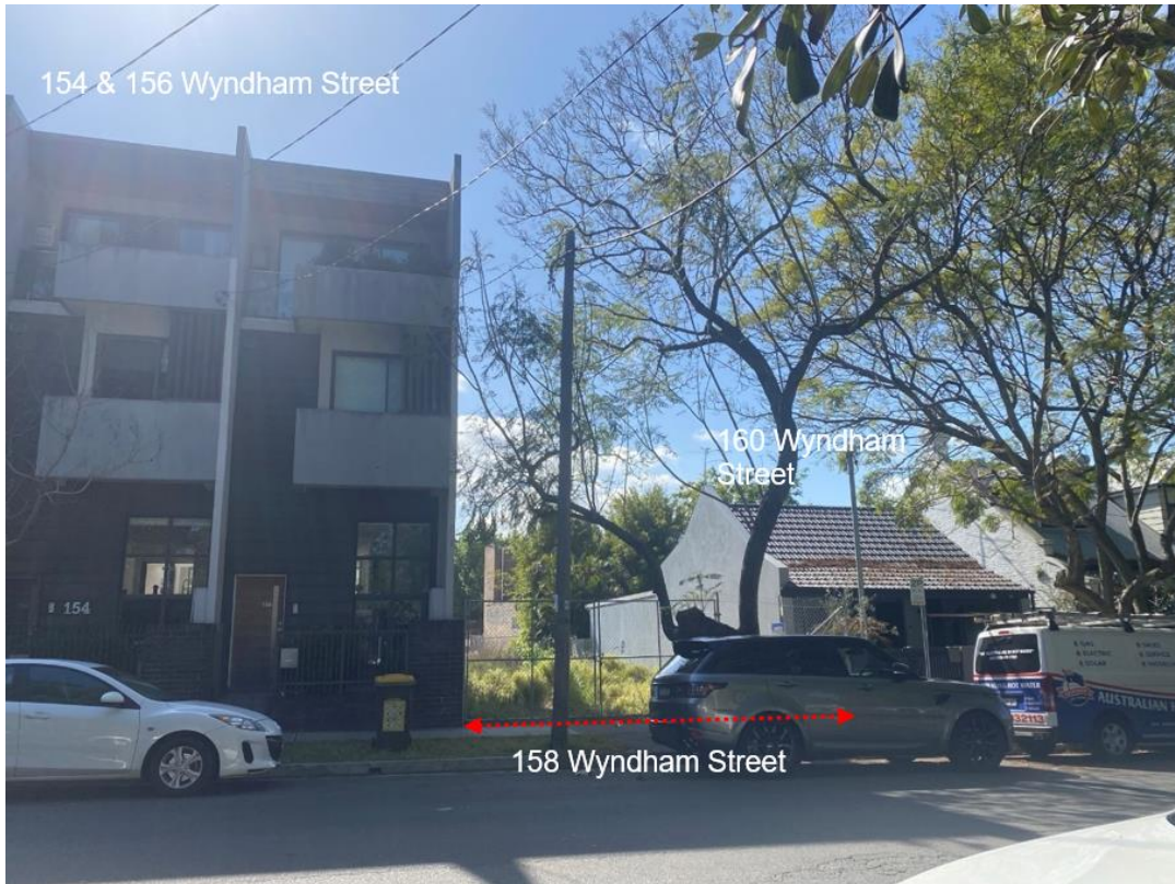
Figure 9: Site viewed from Wyndham Street looking east
